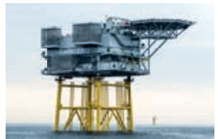
December Green energy for 3 million households thanks to the offshore wind substations in the North Sea.
